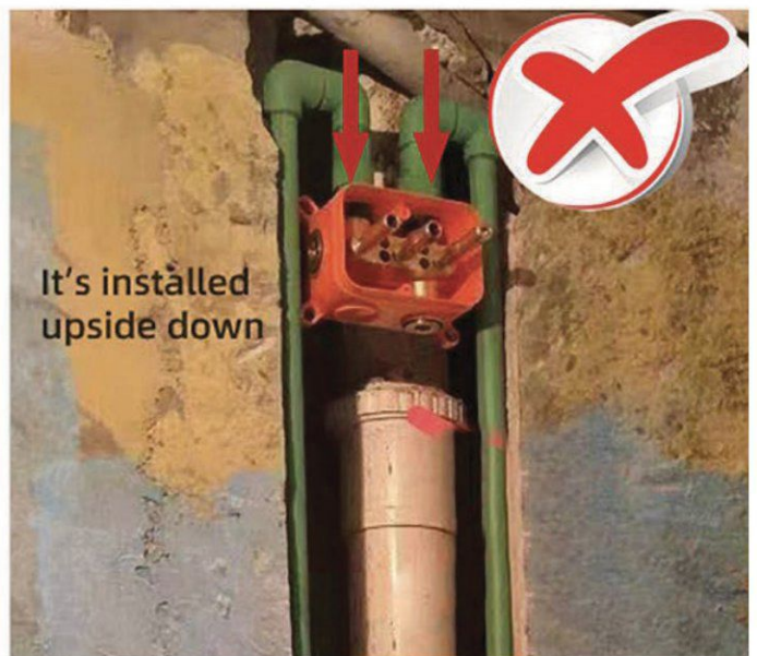
The installation of concealed plastic box in wrong way
